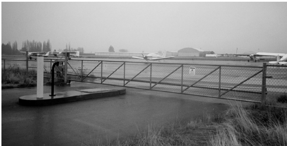
Access Road & Electronic Gate at North Apron
