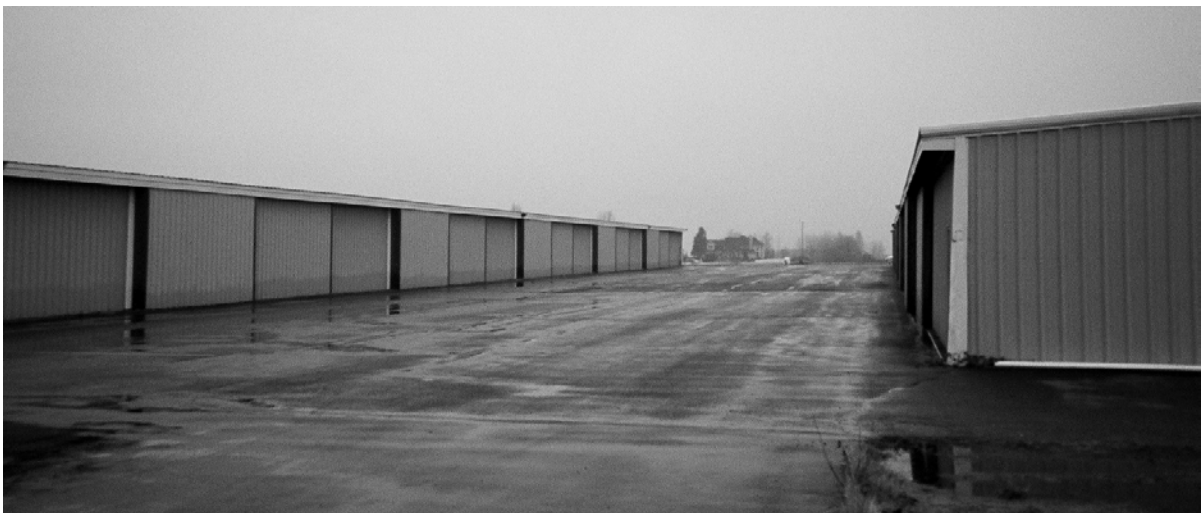
Airport Hangars (North)
