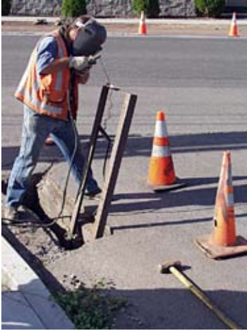
Drainage grate repair
