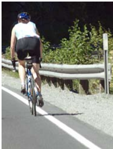
A road without a paved shoulder leaves the bicyclist with little maneuvering space and can discourage all but the most experienced riders
