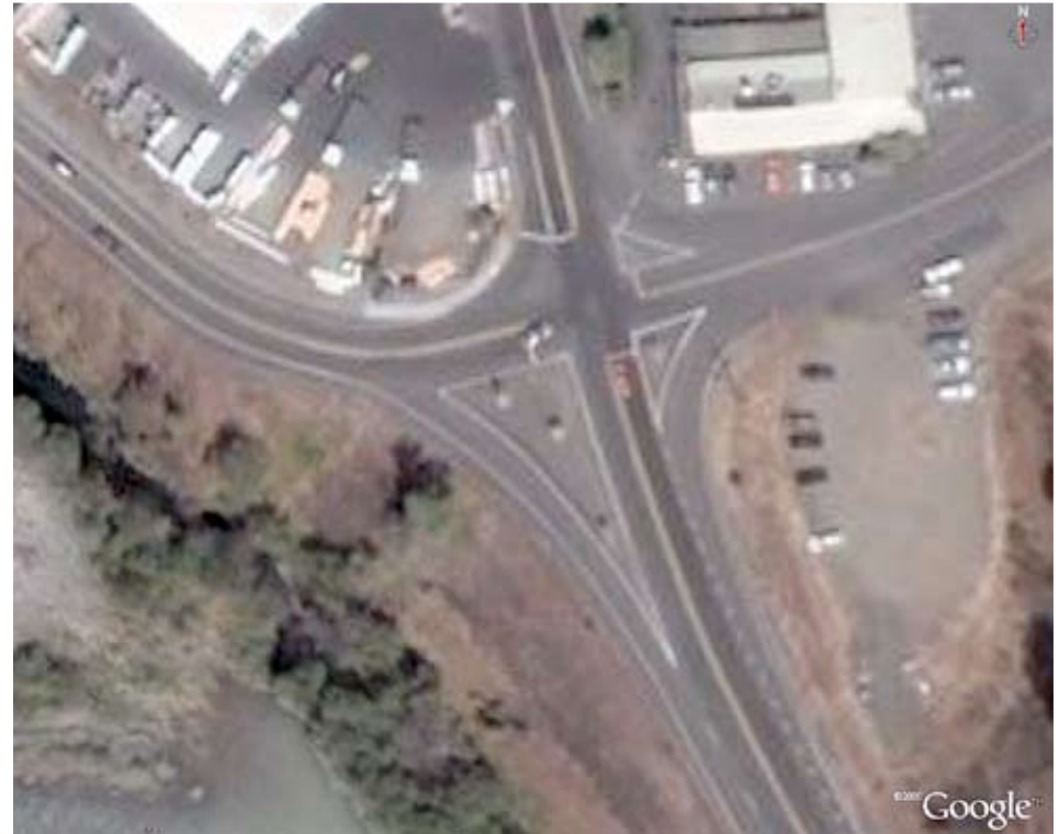
Existing intersection with slip lanes can be difficult for a bicyclist to negotiate. A signal would potentially increase crossing distance and conflicts.
