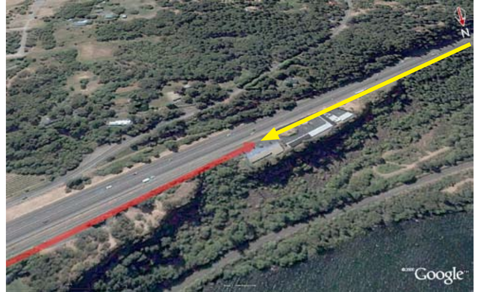
Westcliff Dr. project (red) and HCRH project from Mitchell Point (yellow). Abandoned Meredith Motel at west end of road.
