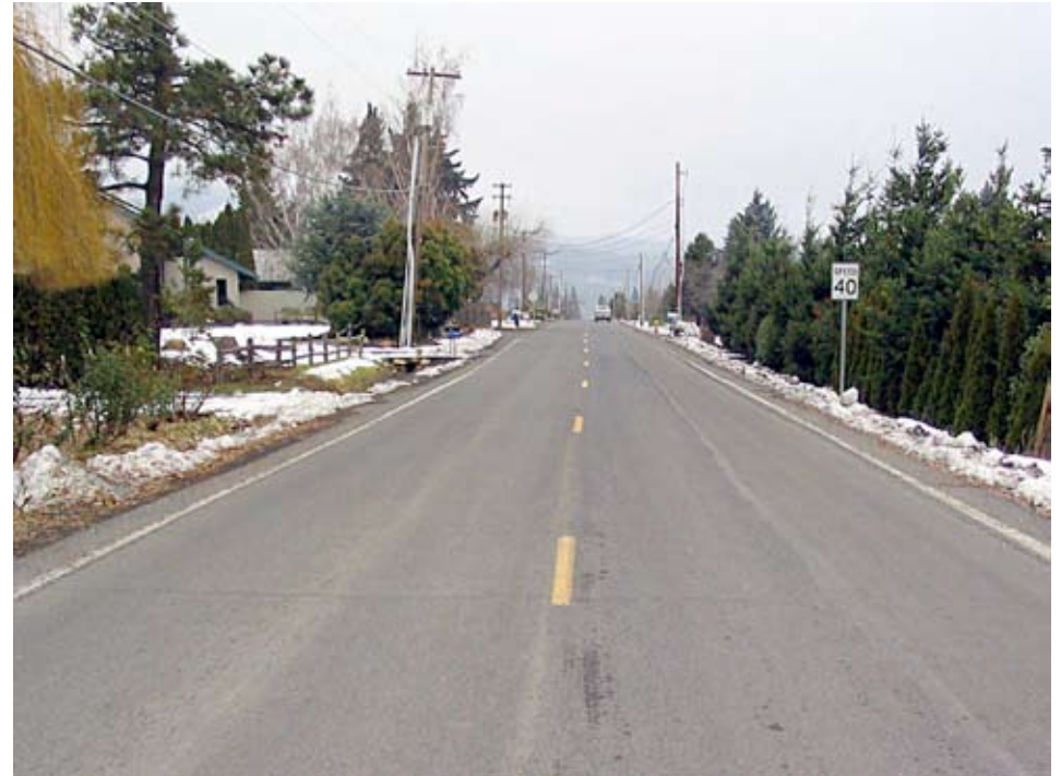
Looking north at Fairview Dr.
